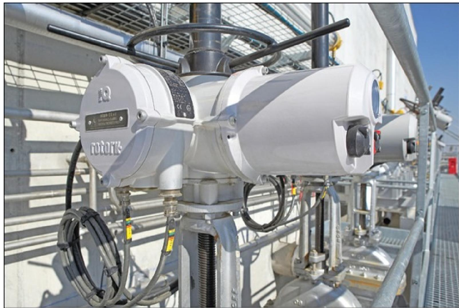
**Figure 10.1.a.** Electric actuator with direct mounting to the flange of a gate valve.
