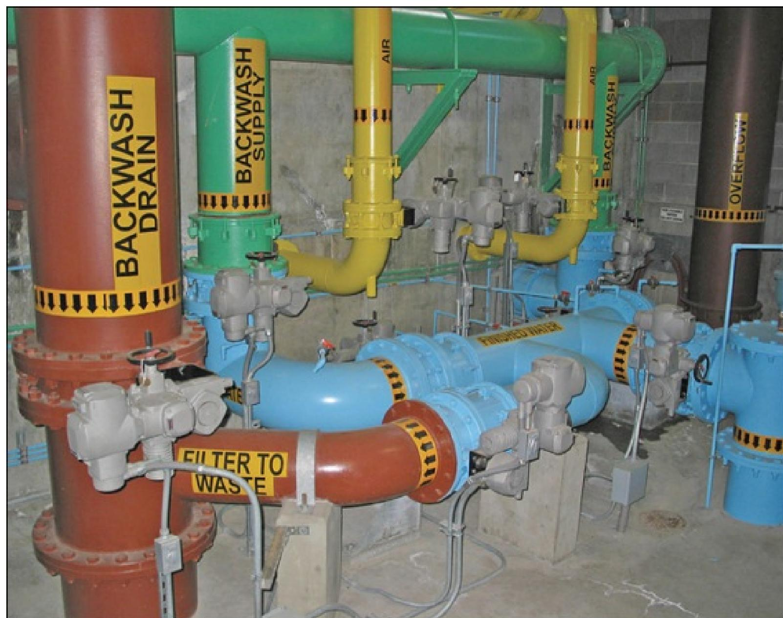
**Figure 13.2.d.** Automated valves for backwash control.
