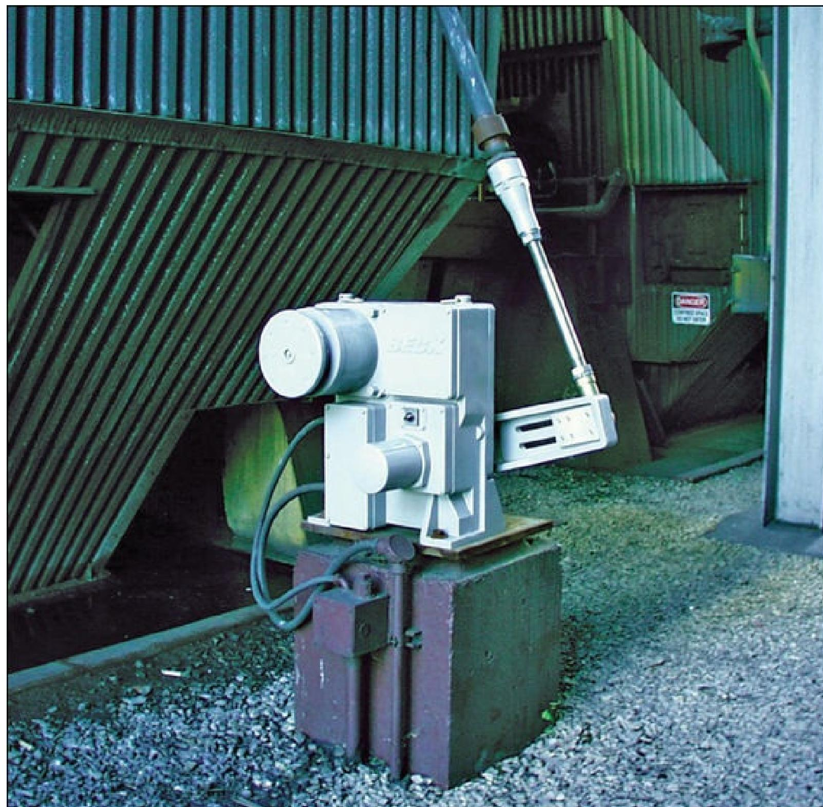
**Figure 13.1.f.** Electric actuator on a damper drive application.
