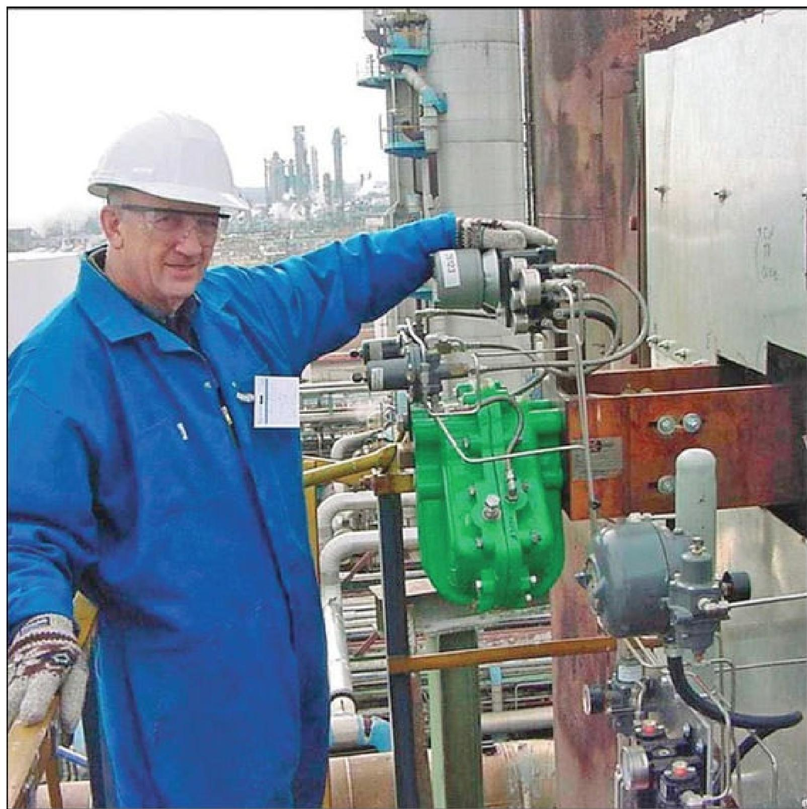
**Figure 12.1.a.** Fluid power actuator maintenance.
