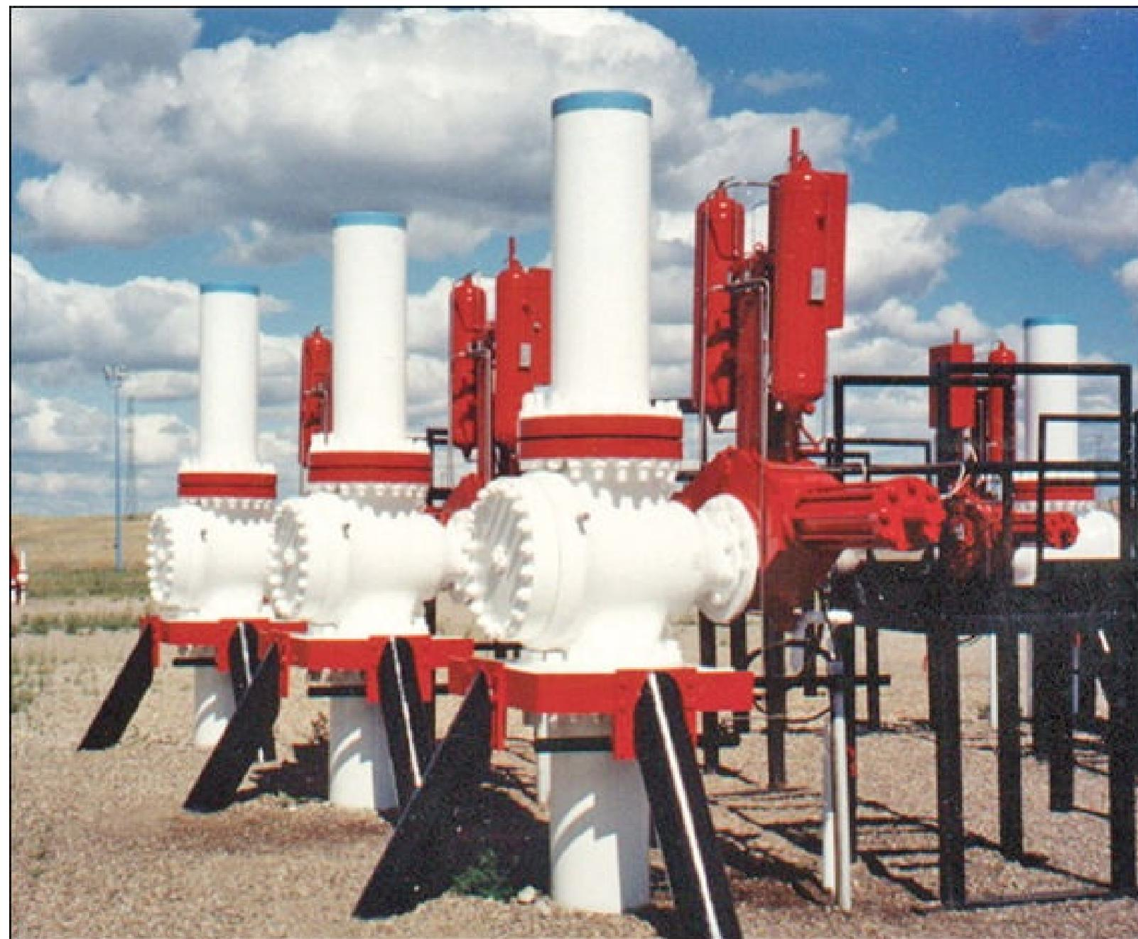
**Figure 13.4.3.a.** Valves on gas pipeline tapered plug valves.
