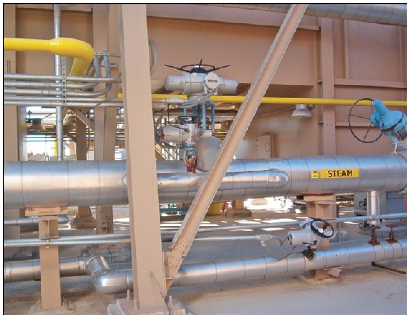
**Figure 13.1.c.** Electric actuators on steam lines in a power plant.
