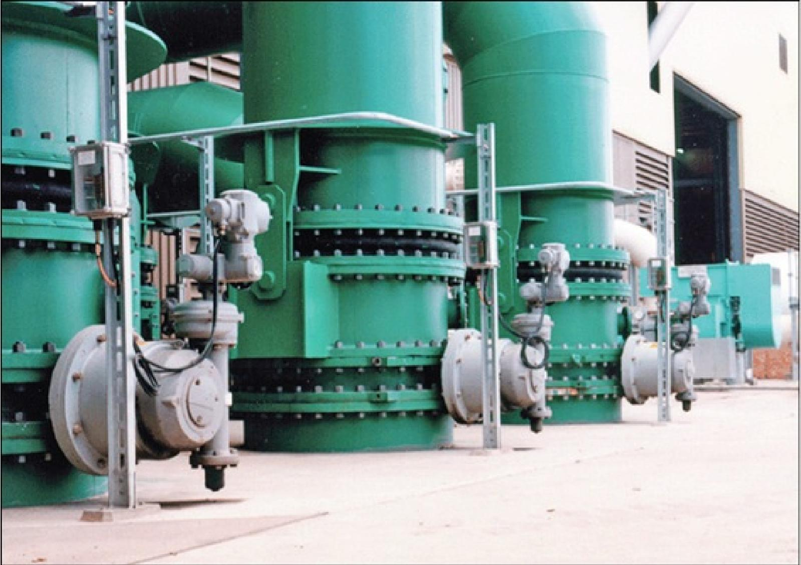
**Figure 6.1.1.2.a.** Large electric multi-turn actuators with secondary quarter-turn gearbox on butterfly dampers. *Image courtesy of Auma.*
