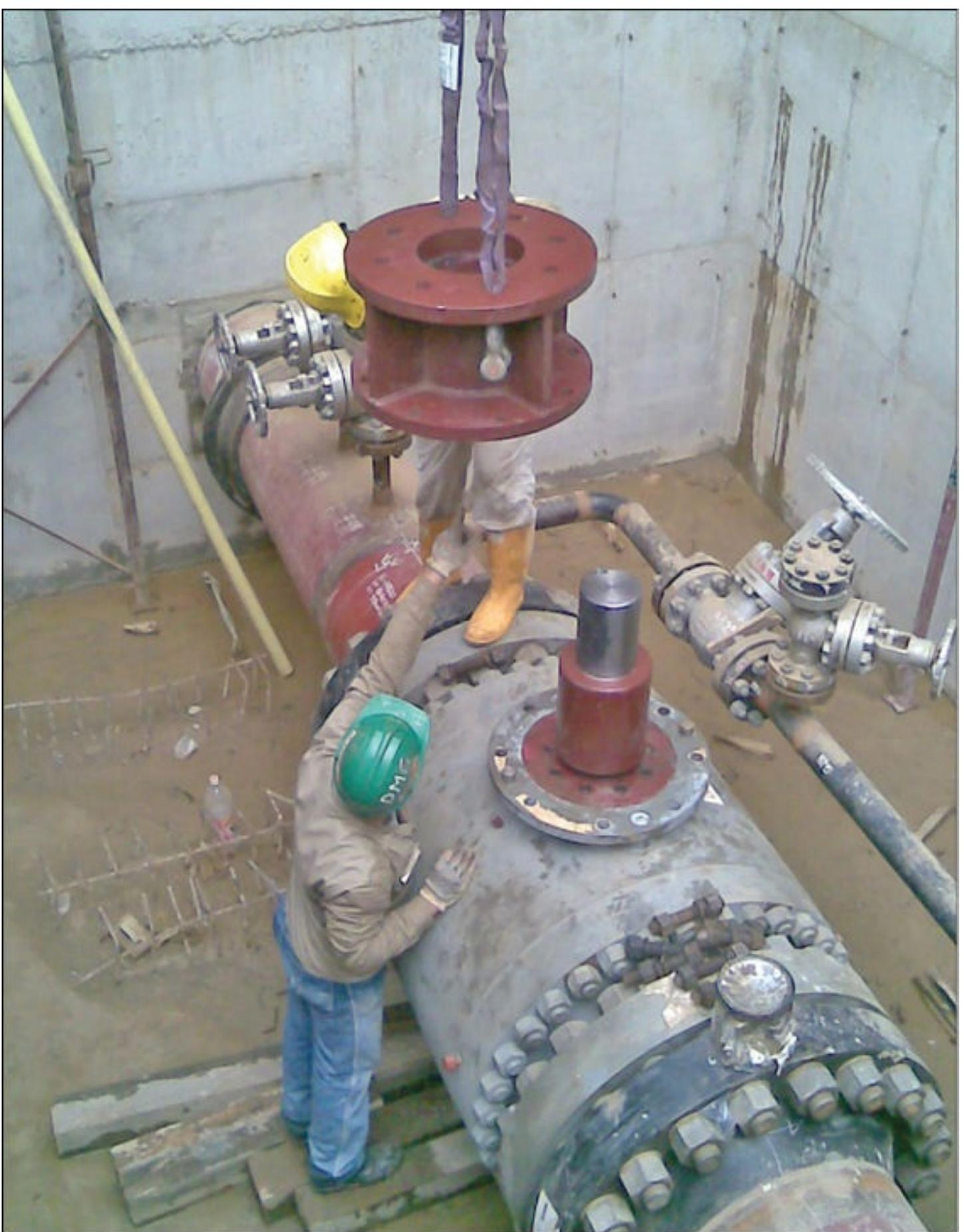
**Figure 11.3.2.a.** Mounting hardware for a ball valve retrofit. The static spool piece is on the sling and the dynamic stem coupling is on the valve stem.
