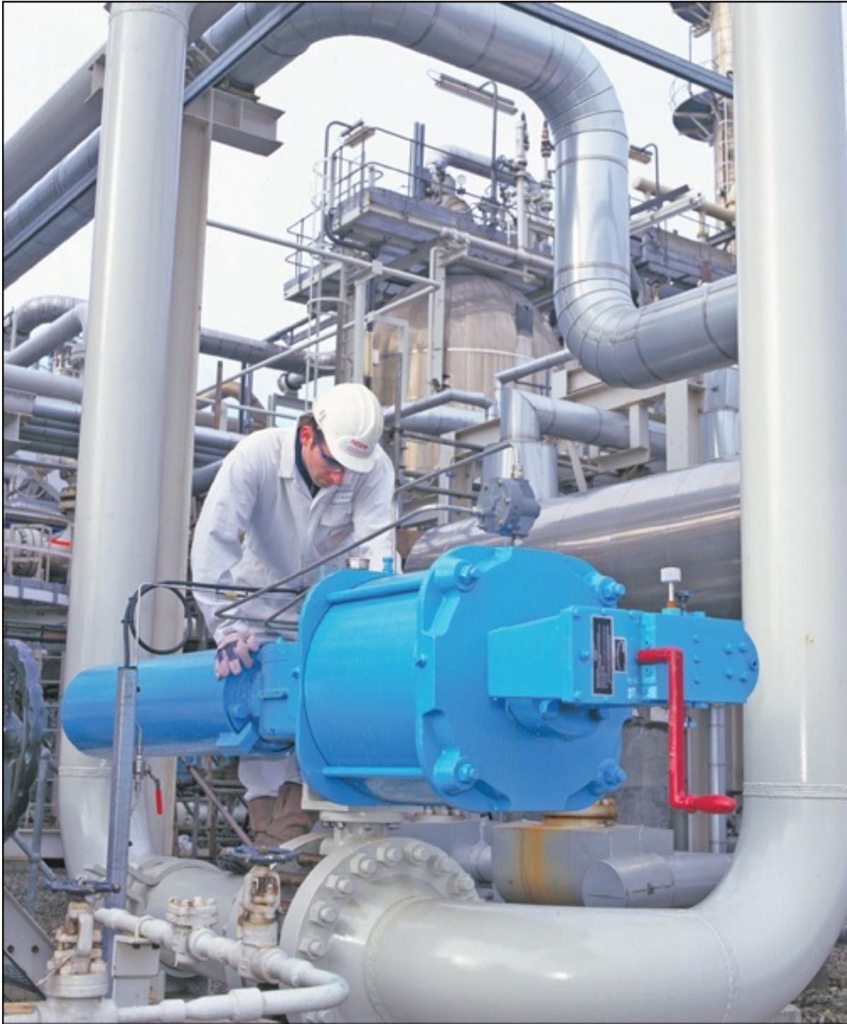
**Figure 5.5.b.** Spring return pneumatic actuator with hydraulic manual override (red handle).
