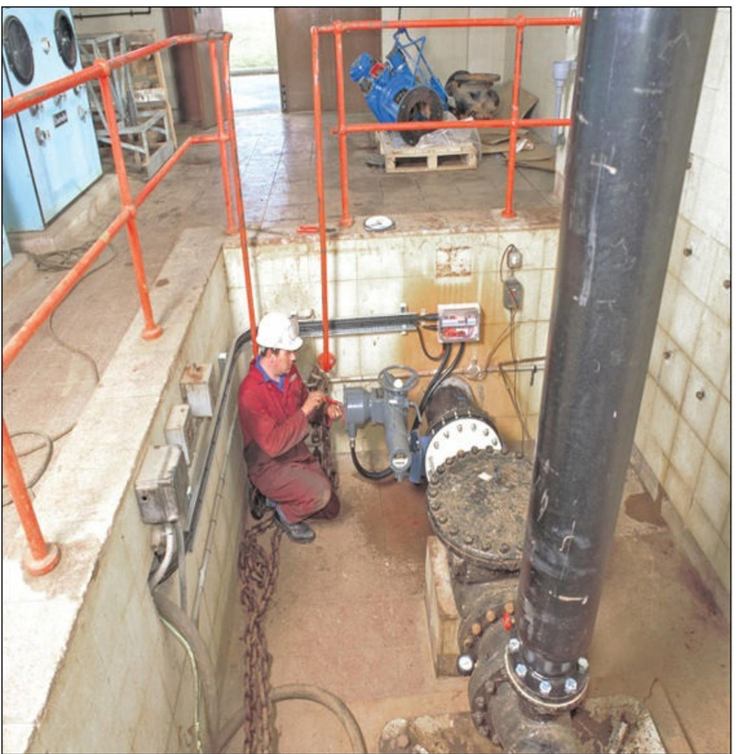
**Figure 11.1.b.** New electric actuator being retrofitted to a valve in an existing plant. *Image by permission of Rotork®.*
