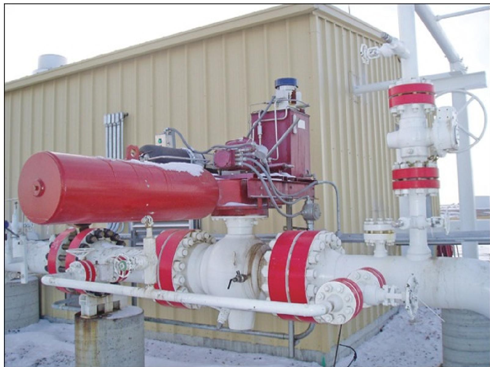
**Figure 6.3.c.** Large electro-hydraulic actuator on a pump station ball valve.
