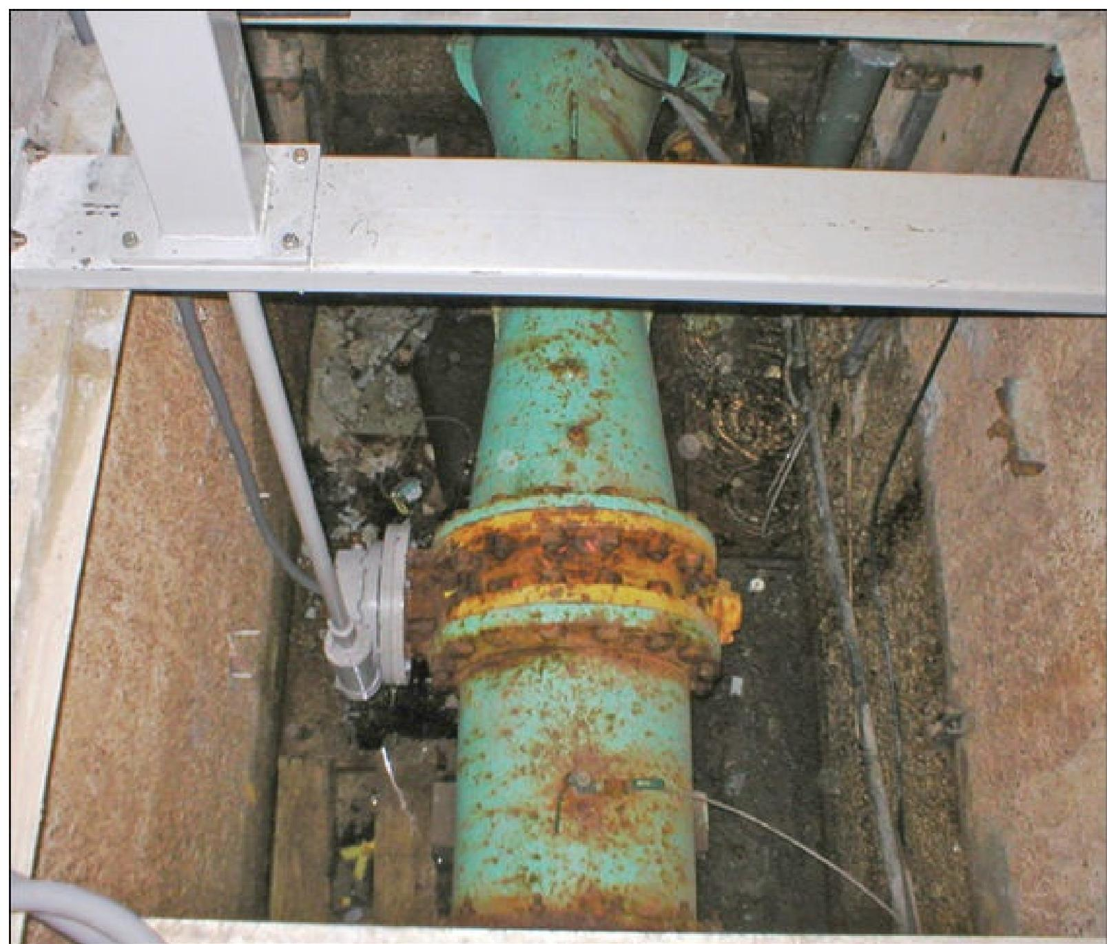
**Figures 11.3.2.b.c.d.** In this application an old water-powered actuator on a butterfly valve in a pit was replaced with a new electric actuator. Due to space restrictions, a compact quarter-turn gearbox was located on the valve stem and a drive shaft was connected to a multi-turn actuator at grade level to drive the gearbox.
