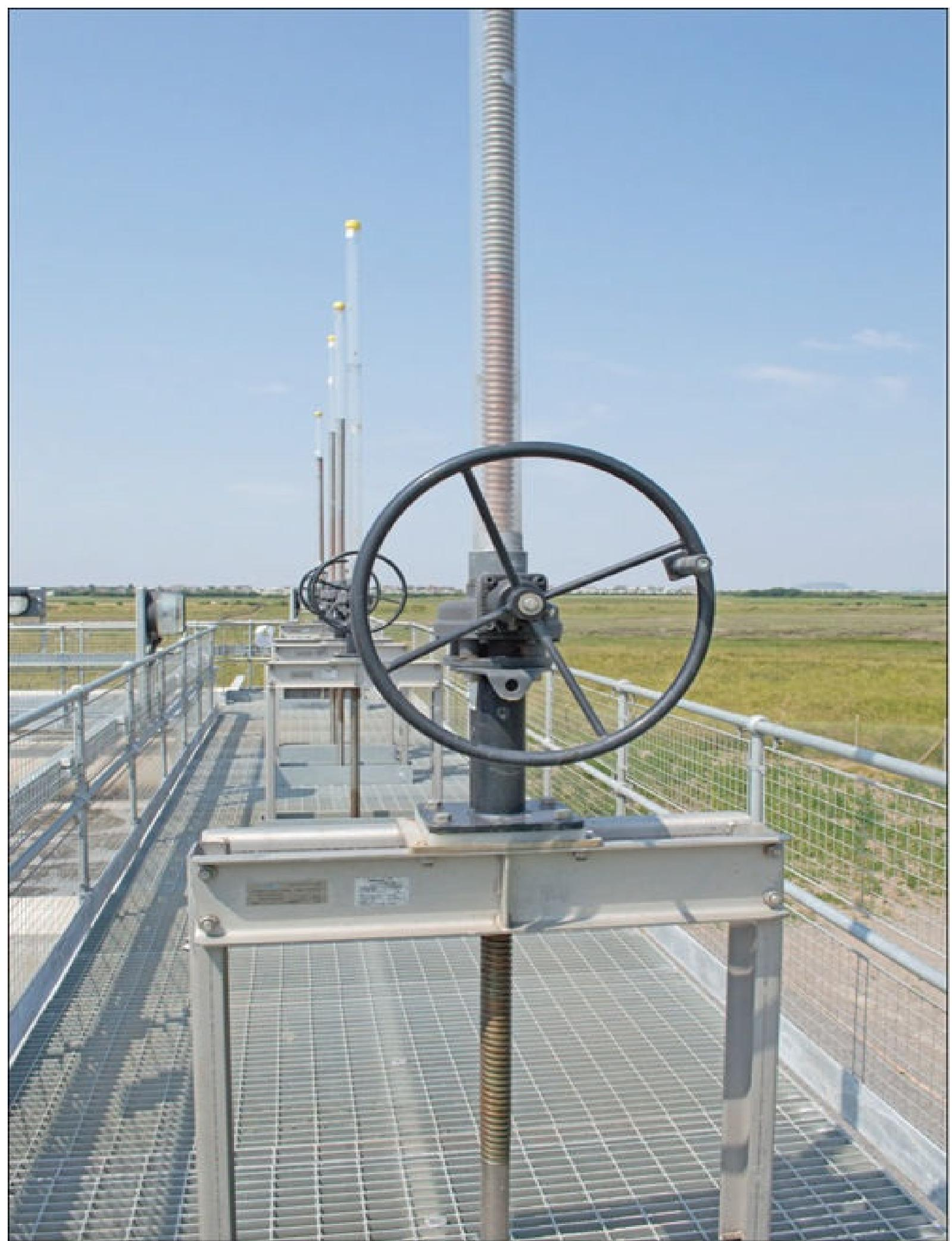
**Figure 5.1.a.** A sluice gate with a long stem, vulnerable to buckling if overloaded
