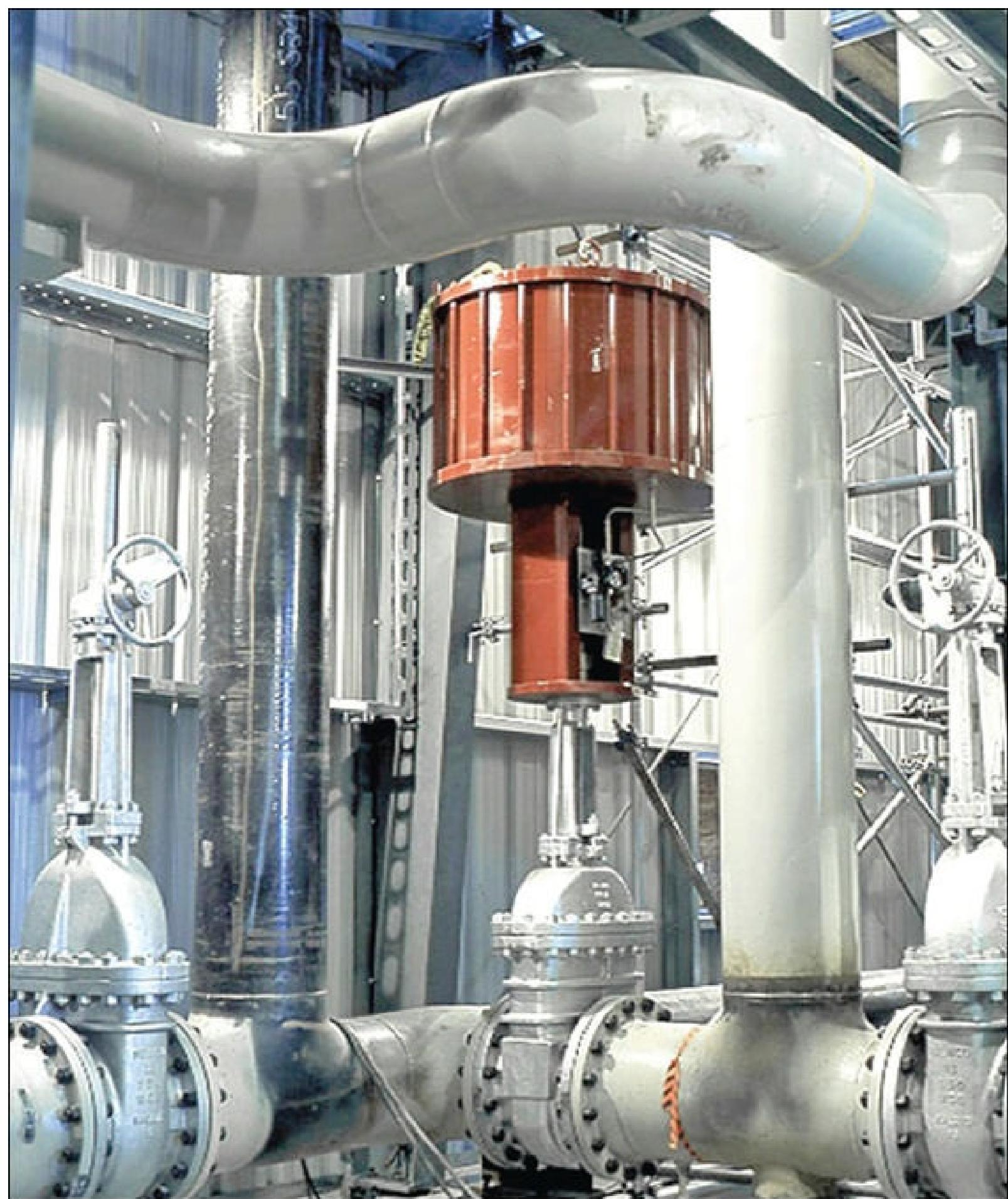
**Figure 6.2.1.3.a.** Large fluid-powered double-acting linear actuator on a gate valve.
