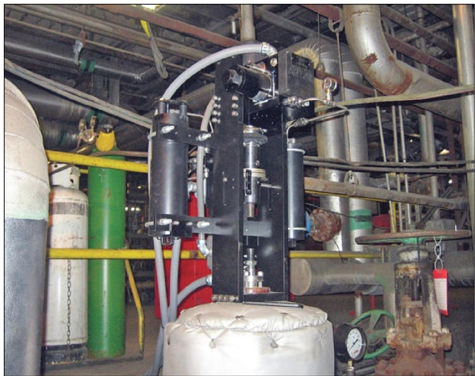
**Figure 6.3.a.** Electro-hydraulic actuator on a boiler feedwater recirculation valve.
