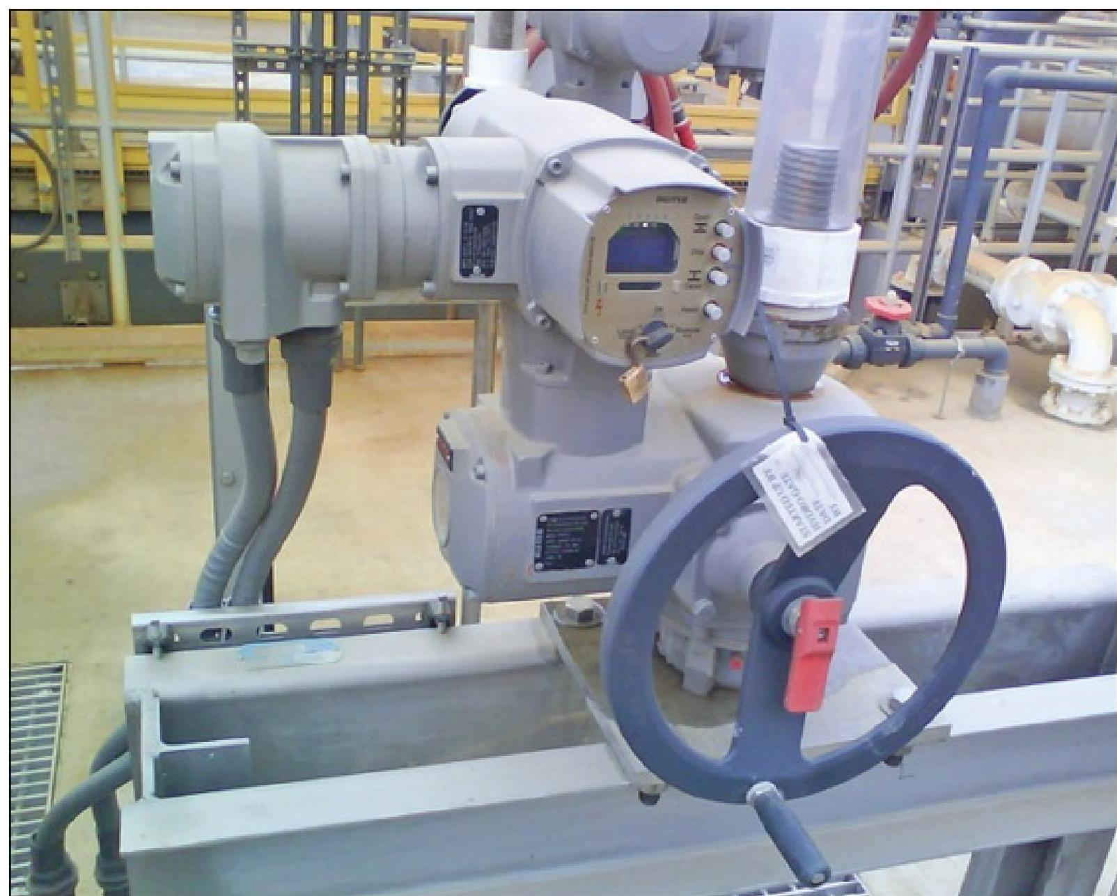
**Figure 6.1.1.1.a.** Multi-turn electric actuator on a sluice gate.
