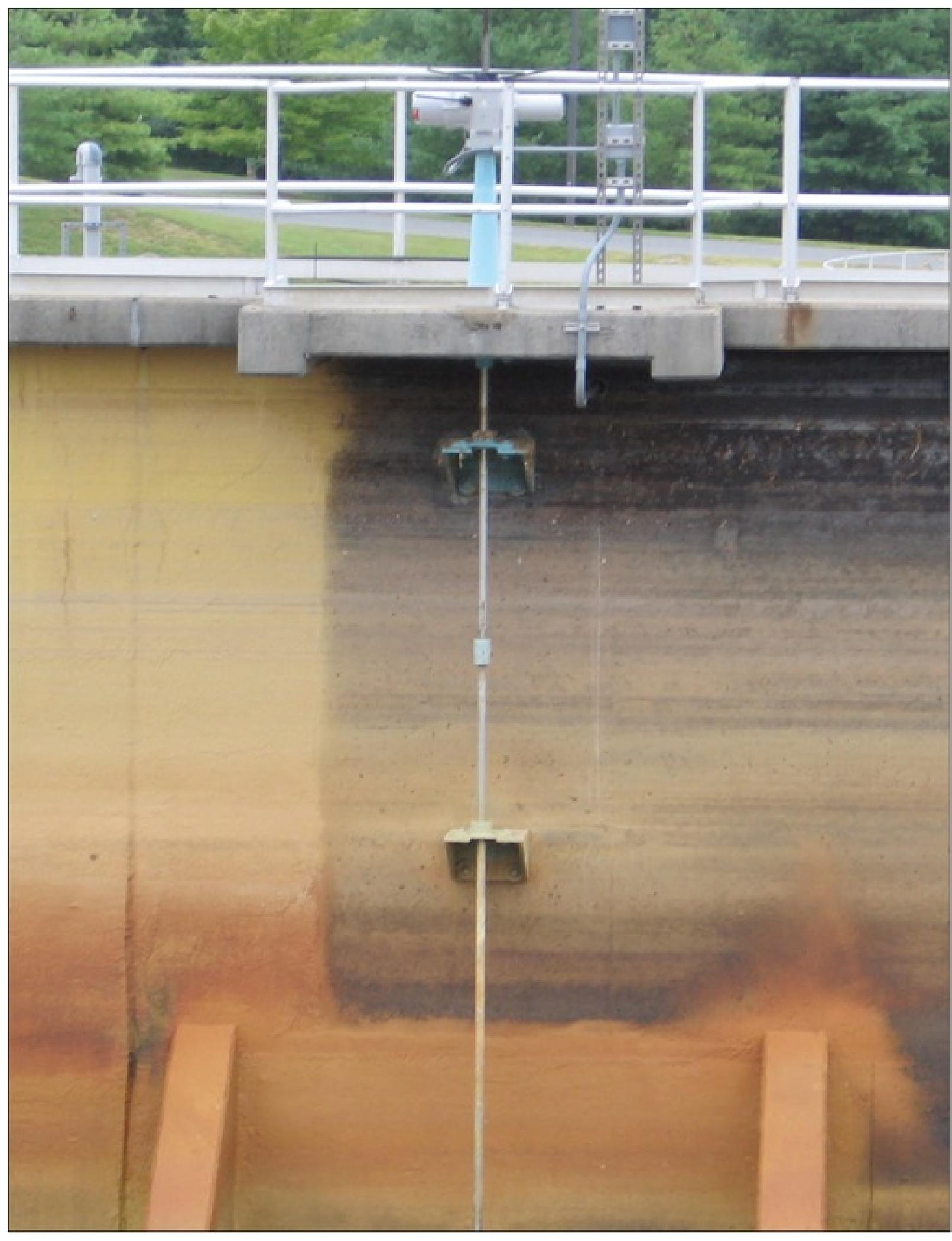
**Figure 14.2.a.** Motorized sluice gate with extended stem. Note the stem guides to reduce buckling risk. *Image by permission of Rotork®.*
