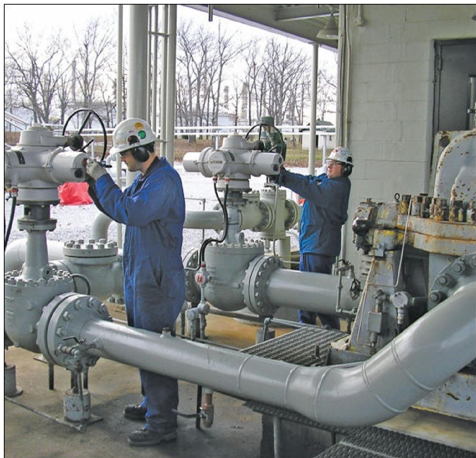
**Figure 12.2.a.** Electric actuator maintenance.
