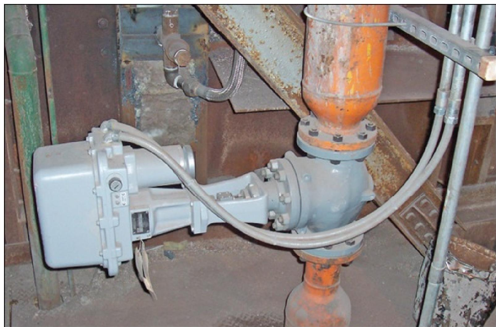
**Figure 6.1.2.3.b.** Electric linear valve actuator mounted on a sliding stem control valve.
